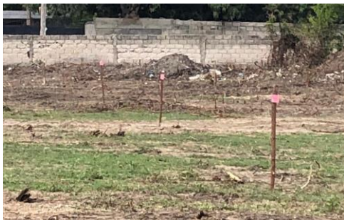
Housing lots being marked on the site for Village Dominique.
